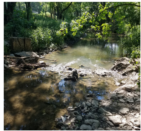
↑ Cross vane weir on the Phinney Branch in Champaign, Illinois.
