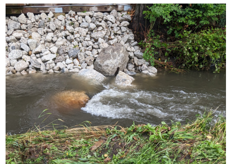
↑ J-hook structure under high flows after a stabilization project in Urbana, Illinois.
